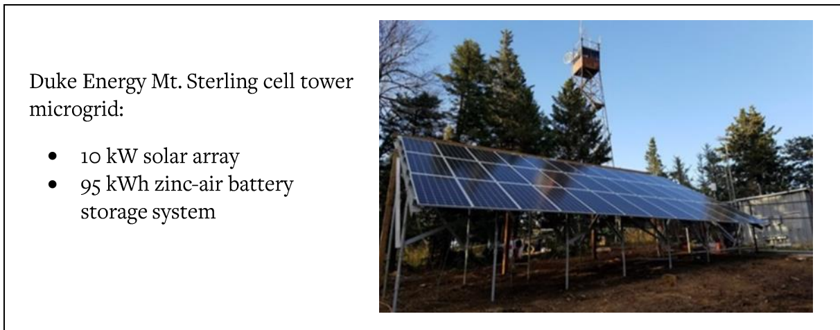
Figure 3. Duke Energy cell tower installation on Mt. Sterling 27
