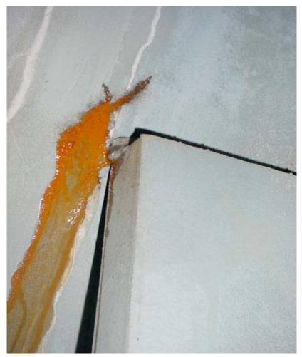
As a result of questions during the ACRS discussion period relating to BWR thick containment designs like the through wall cracks at Hatch 1 and 2, Fairewinds researched additional failures and found that the Fitzpatrick nuclear power plant developed a large though-wall leak that was not due to corrosion. Once again, here is a unique violation of the BWR containment system that is directly applicable to the Westinghouse design of the AP1000.
