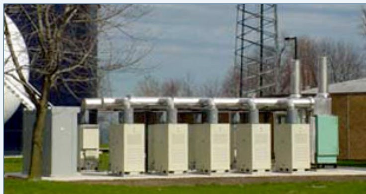
Utility-financed CHP: Five of the ten microturbines installed and financed by Alliant Energy at the Sheboygan Wastewater Treatment Facility in Sheboygan, WI. Photo: ACEEE
