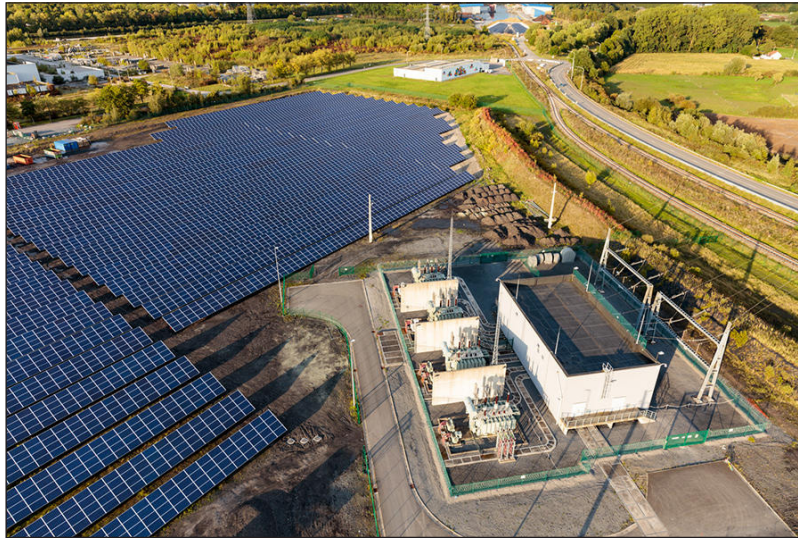
Figure 7. Rooftop Solar Serving a Data Center 104
