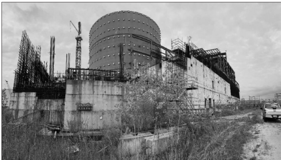
Figure 4. The Cancelled, Partially Built V.C. Summer Nuclear Plant 50
